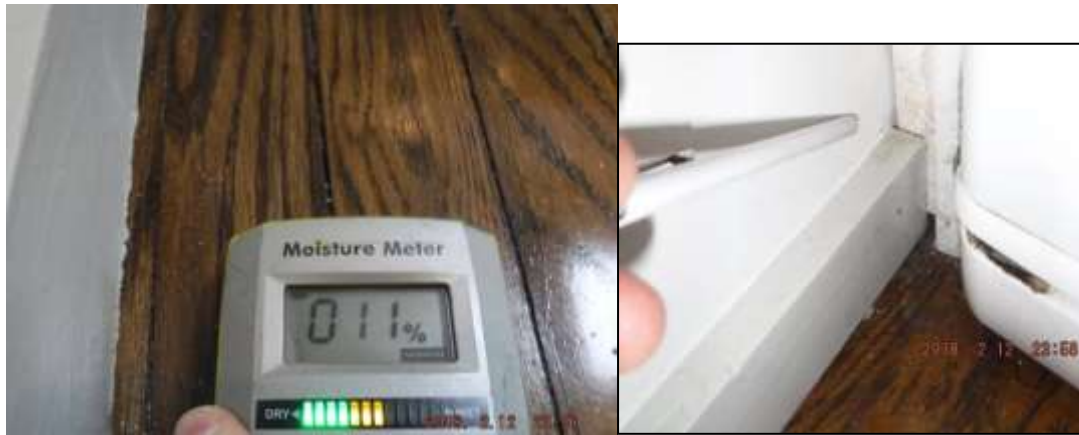
Figure 11 Example of active moisture and dark water stains on wood floor in kitchen adjacent to the bathroom and roof & skylight leaks. Recommend a building contractor determine all water/leak sources and advise on repairs before closing.
