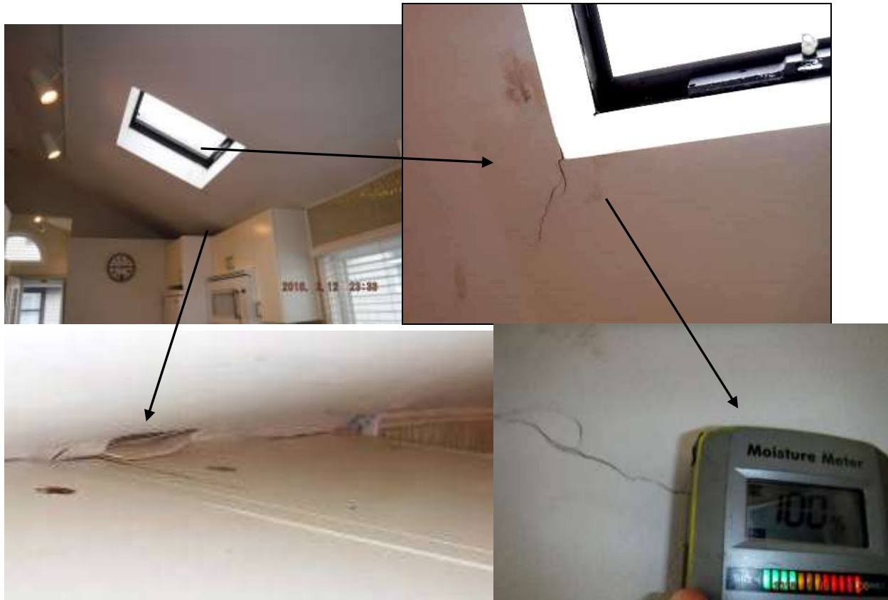
Figure 11 Example of active moisture and dark water stains on wood floor in kitchen adjacent to the bathroom and roof & skylight leaks. Recommend a building contractor determine all water/leak sources and advise on repairs before closing.
